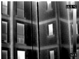
Thermal bridges are easily identifiable through infrared thermography: the different characteristics of materials give to each structural element a different temperature.
