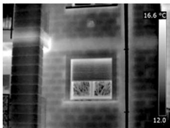
The different thermal resistance of mortar and bricks allows the professional operator to clearly recognise the wall texture, despite the covering plaster.
