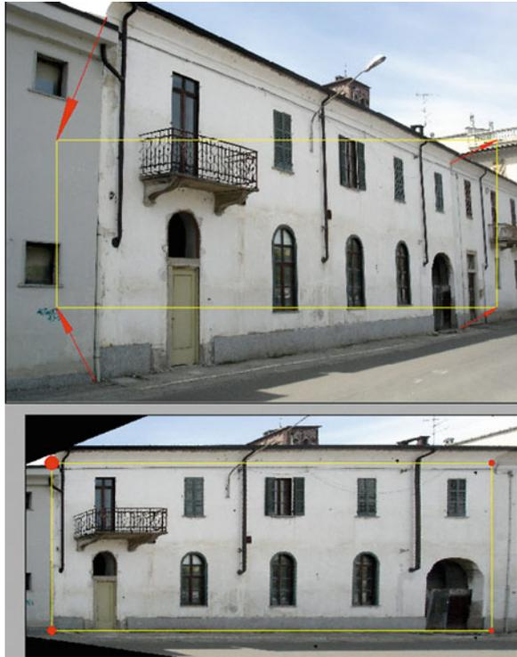
The accuracy achievable in the measurements performed on the plane that is chosen for the straightening can vary within very wide limits, depending upon several parameters:
