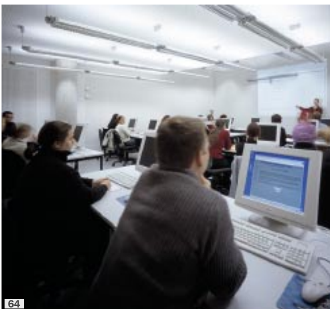
Lighting management systems permit control and regulation of individual groups of luminaires. Room lighting thus remains adequately bright while the presentation area lighting is dimmed (Fig. 64).
