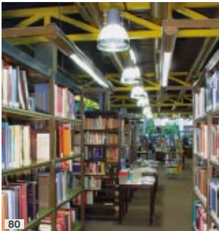
Shelf unit lighting with asymmetrical wallwashers heightens vertical illuminance. Book titles and colours are thus more readily identifiable.
