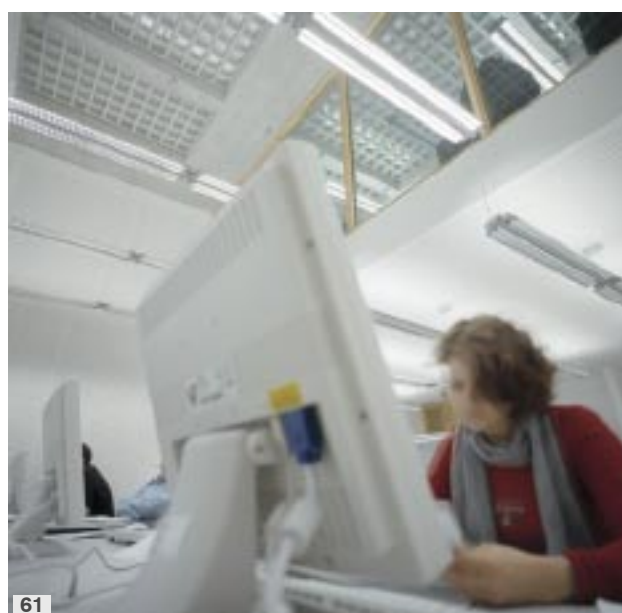
At computer workstations, luminaires need to be well shielded to prevent reflections being cast onto screens and ensure that colours are rendered accurately and screen brightness is maintained. (Fig. 61).
