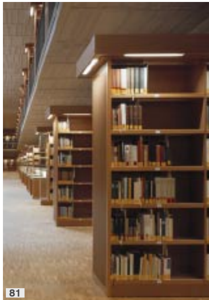
Shelf unit lighting with asymmetrical wallwashers heightens vertical illuminance. Book titles and colours are thus more readily identifiable.
