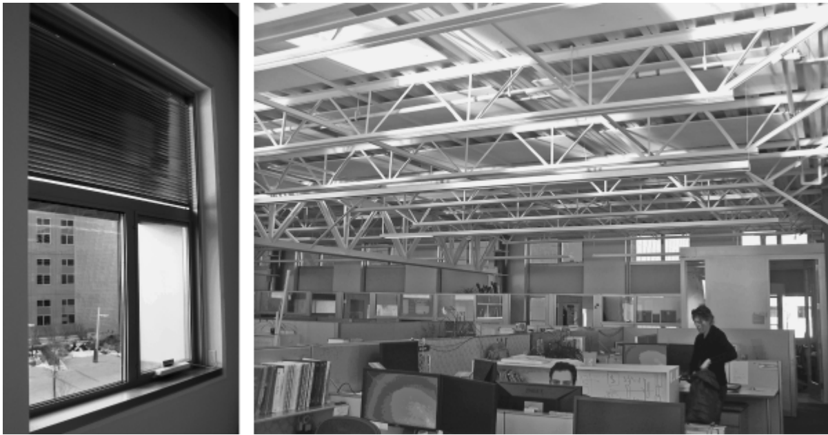
Fig. 4.21 National Renewable Energy Laboratory (NREL) Research Support Facility (RSF): window with fixed louvers on top half (left) and the resulting upward-reflected daylight on the ceiling of the office space (right)
