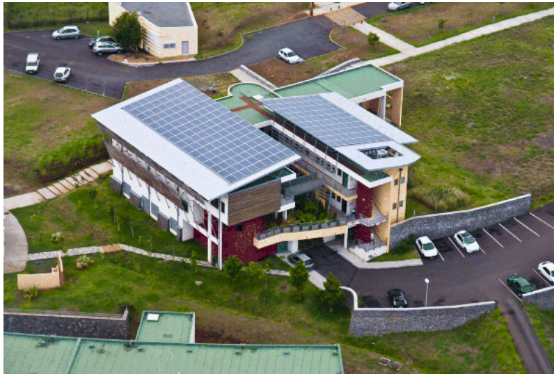
Fig. 7.72 ENERPOS building on Reunion Island. BIPV roof: 365 m 2 of PV panels to balance the low consumption of the building (Photo courtesy of Jérôme Balleydier)
