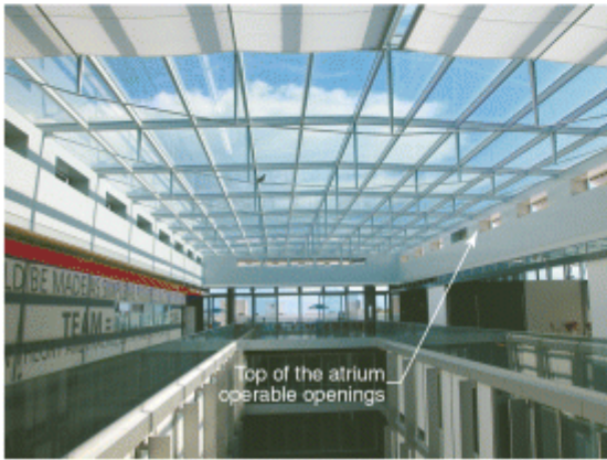
Fig. 4.3 Natural ventilation in an atrium (BC-EPFL Lausanne Switzerland, Architect: R. Luscher Lausanne, Energy Concept: Sorane S.A, Ecublens)
