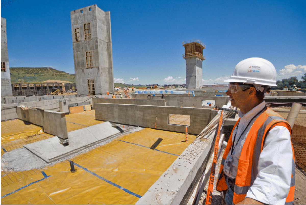
Fig. 7.52 Thermal mass “labyrinth” during construction (Image courtesy of Pat Corkery, NREL)
