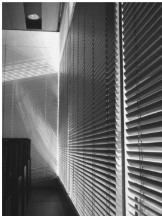
Fig. 4.18 Reflected sunlight from Venetian blinds that are designed to protect occupants from direct solar radiation while reflecting it onto the ceiling to provide diffuse daylight
