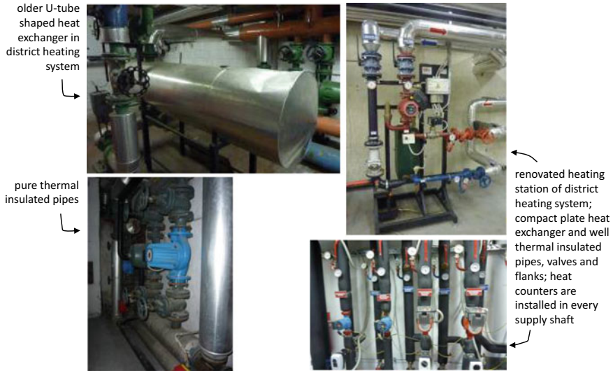
Fig. 8.45 Renovation of district heating station decrease heat consumption in multi-family buildings up to 20%
