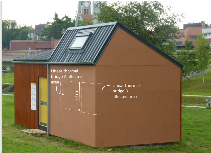
Fig. 3.11 Photo of Virtual Lab building with impact area of analysed thermal bridges
