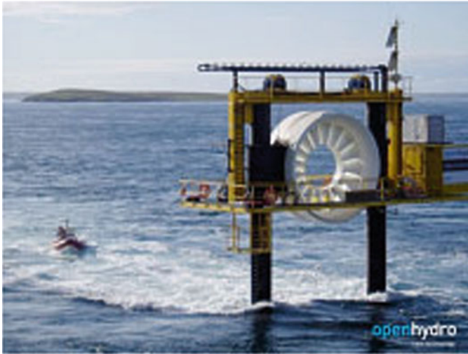
Fig. 2.13 Tidal current can be utilized by underwater turbines (Whole Building Design Guide, www.wbdg.org/resources/oceanenergy.php )
