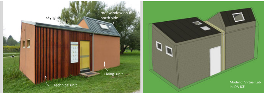
Fig. 1.13 Photo of Virtual Lab building (left), Virtual Lab building in computer simulation tool IDA-ICE (right)
