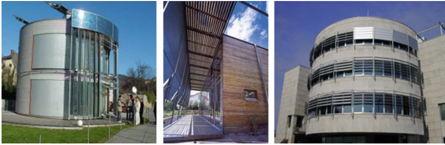
Fig. 3.16 Examples of adjustable, high solar reflective shading devices; rotating shading louvers with integrated PV modules for electricity production (left), shading roll installed in the way that enable double side convection cooling and daylighting of interior of the building (middle), adjustable reflective shading fins installed 25 cm in front of the facade (right), in presented cases, total solar irradiation transmittance (including shading and window glazing) is below 0.08
