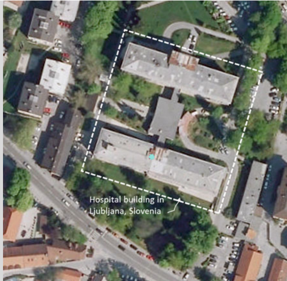
Fig. 13.5 Hospital building in Ljubljana, Slovenia (gis. arso.gov.si/atlasokolja)
