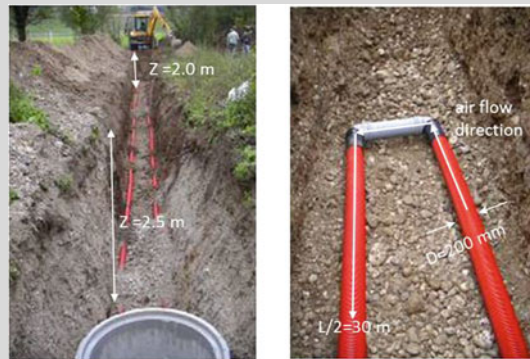
Fig. 11.36 U-shaped ground heat exchanger
