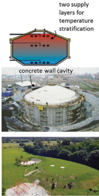
Fig. 8.11 Examples of long-term water (left) and pit-type seasonal heat storage (right) (SDHplus 2015)
