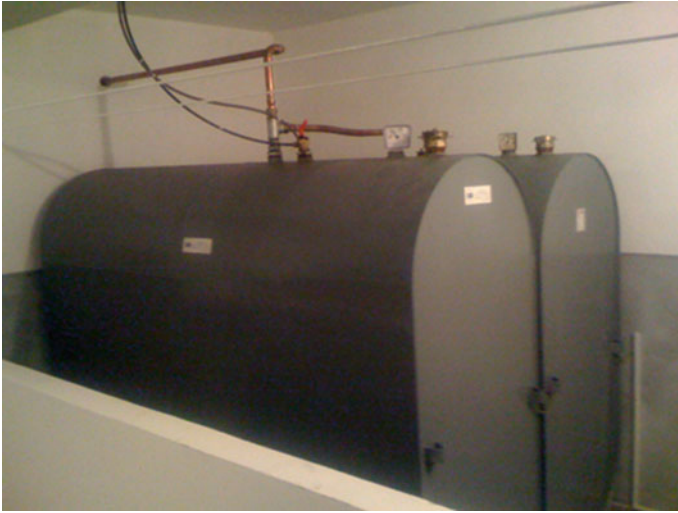
Fig. 2.18 Reservoirs for lightweight heating oil must be placed in a watertight pool to prevent the leakage of oil into ground water or must be made as double wall tanks with integrated leakage sensors
