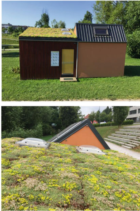
Fig. 3.5 Green building structures improve the microclimate in urban environments, absorb air pollutants, capture rainwater and reduce heat transfer to building interiors
