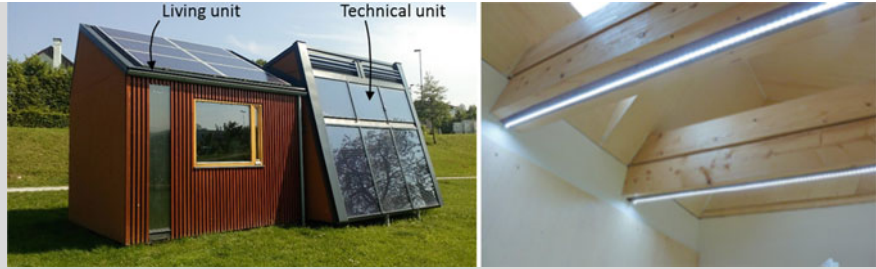
Fig. 12.10 Photo of Virtual Lab building (left), LED luminaires in living unit (right)
