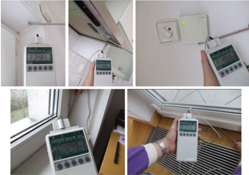
Fig. 4.15 Air velocity at the leaky details on the building envelope is in the range from 2 to 4 m/s and air leaks can be easily detected with air velocity measurement
