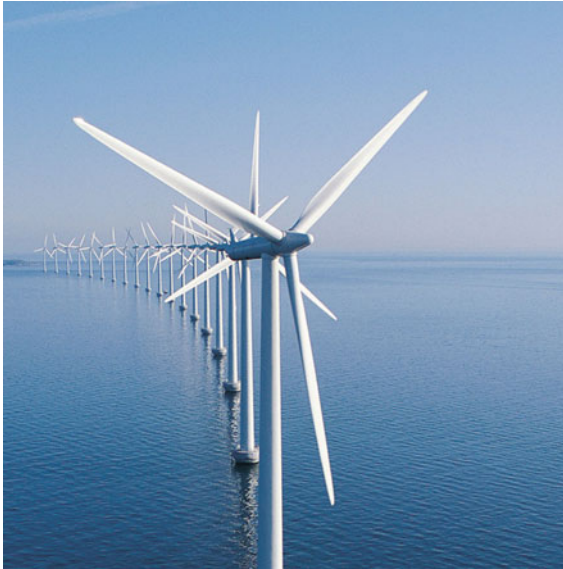
Fig. 2.4 Low energy density is one of the drawbacks of RES; one turbine presented on the picture with rotor diameter of 70 m, has power of electricity generator comparable with mechanical power of the motor of F1 racing car; despite that, electricity production by wind turbines is cost effective especially with off shore applications because of the higher wind speeds in comparison to those on the land ( http://wonderfulengineering.com/38-high-def-wind-turbine-pictures-from-around-the-world/ )
