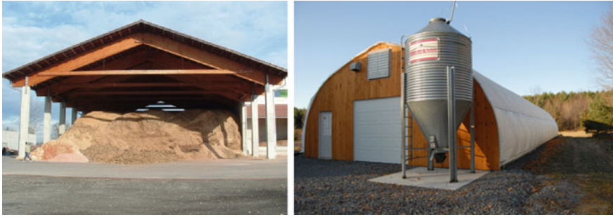
Fig. 2.21 Outdoor storage for wood chips (left); outdoor silos for pellets (right) ( www.mywoodpelletsolution.com )
