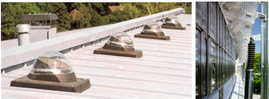
Fig. 1.15 Uniformity of illuminance in day-lit rooms can be improved by skylights and prismatic elements for guiding light toward the ceiling of the room (left: www.solatube.si ; right: www.okalux.com )
