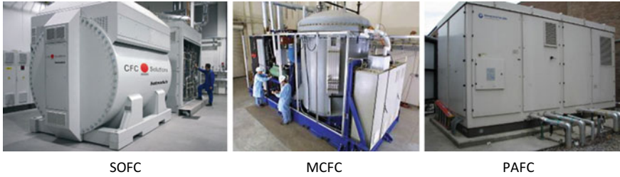
Fig. 7.30 Cogeneration units with different types of fuel cells
