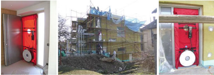
Fig. 4.13 Blower door equipment installed tightly on the entrance door of building (left); it is common practice that the blower door test is performed in new buildings before finishing to enable the airtightness to be improved with minimum cost (middle, right)
