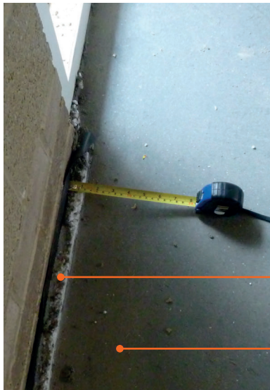
Figure 4.13 Cavities minimum 50 mm clear of debris. Wall tie track system to minimise thermal bridging (right).
