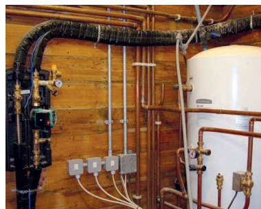
Figure 8.19 Solar thermal system (left).
