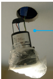
LED downlight with insulation cap
