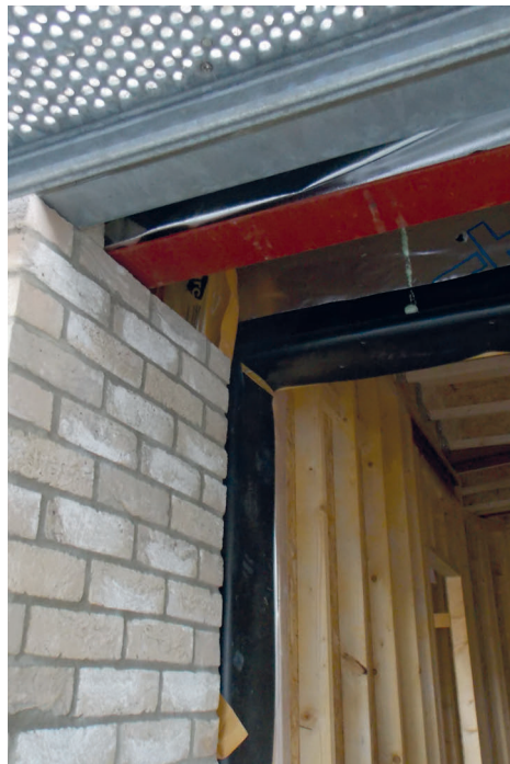
Figure 5.23 Recessed entrance with double steel lintel (left).
