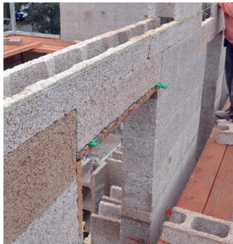
Figure 6.14 External wall ready for concrete pour (right).
