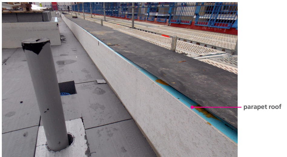
Figure 7.12 Insulation and DPM lining the inside of CLT parapet.
