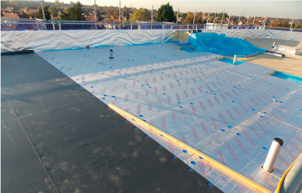
Figure 5.26 Layers of construction on timber flat roof.
