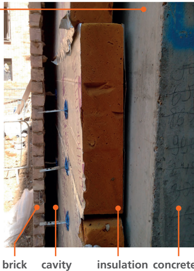
Figure 4.5 Rigid board insulation installed with air gaps.
