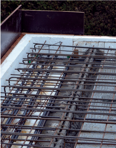
Figure 6.19 Steel bar reinforcement in roof (left).
