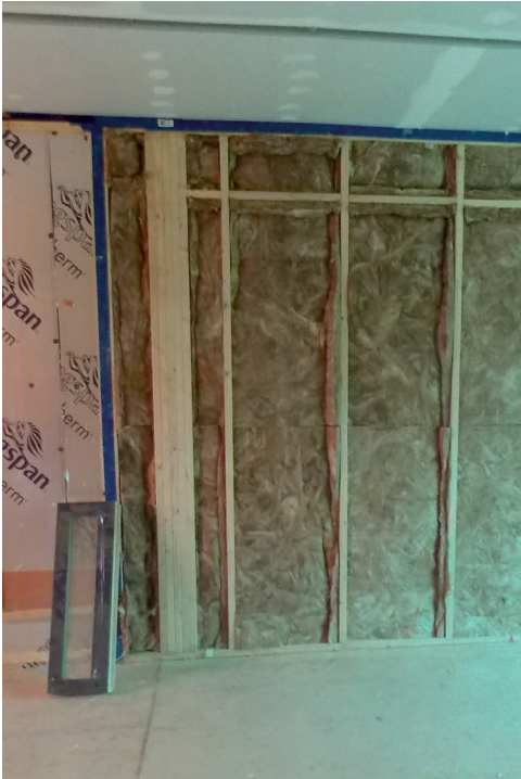
Figure 5.15 Party wall construction (left).
