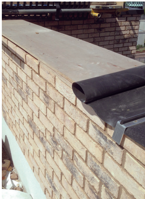
Figure 4.28 a & b Parapet thermal break installed (right).
