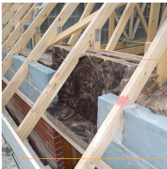
Figure 3.26 Insulation installed before roof finish.
