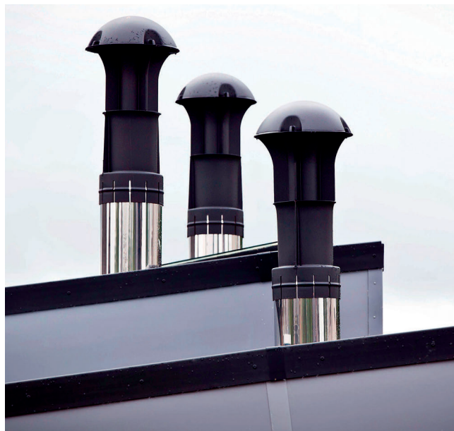
Figure 8.26-28 Passive stack ventilation with heat recovery.
