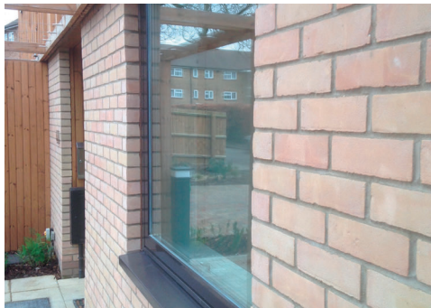
Figure 5.19 EPDM seal adhered to red breather membrane (top right).
