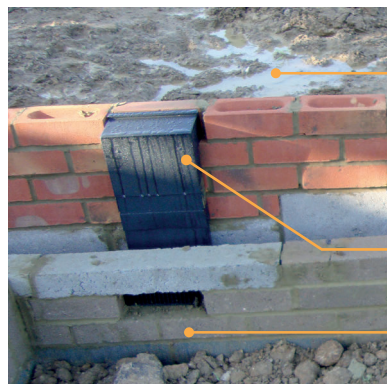
Figure 3.10 Installation of subfloor vents (top left).
