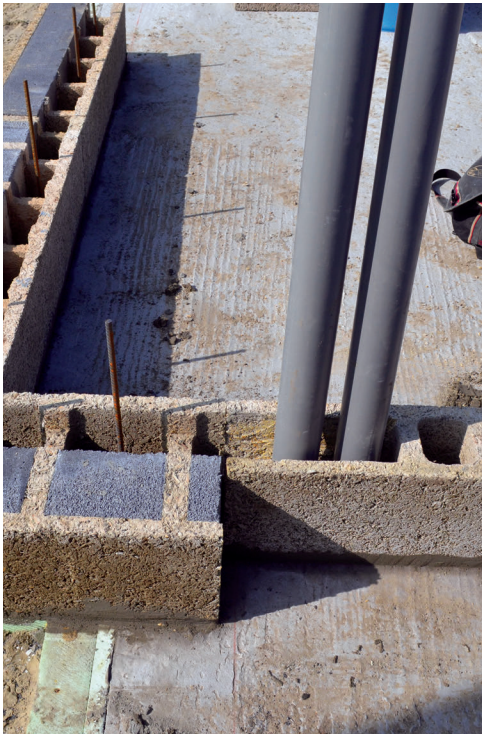
Figure 6.10 Level external door threshold (left).
