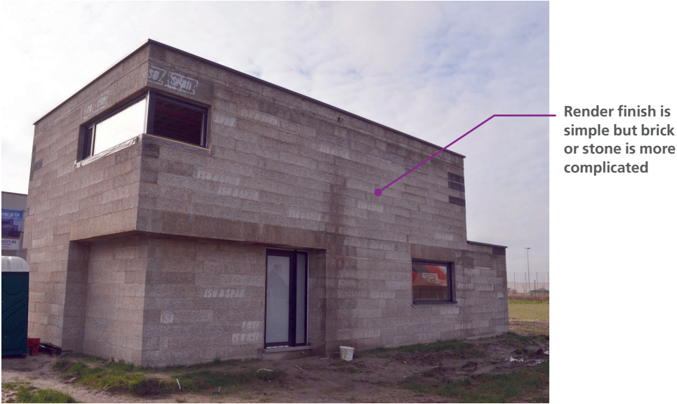
Figure 6.8 ISOSPAN ICF blocks for a house, waiting to be rendered white.
