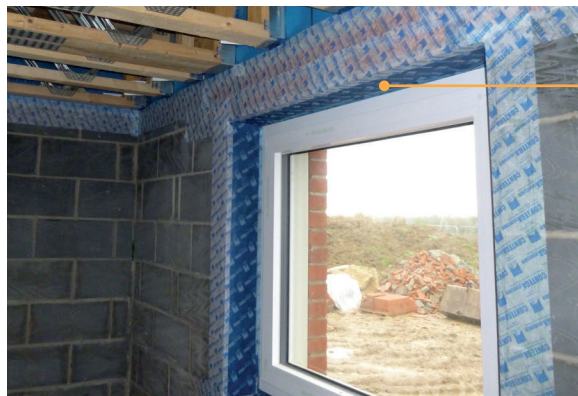
Figure 3.22 Floor joists sealed with airtight membrane and tape.
