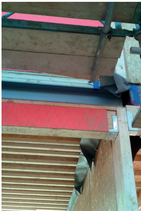
Figure 5.12 Intermediate floor timber cassette (left).
