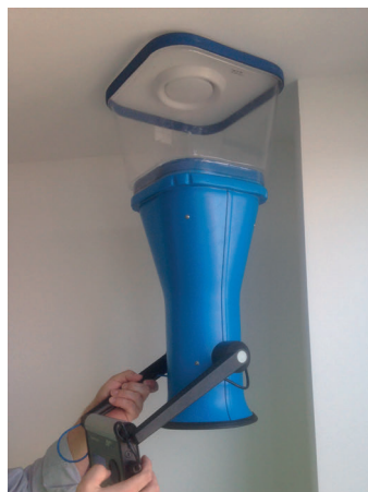
Figure 8.6 Flow rate test to commission fans.
