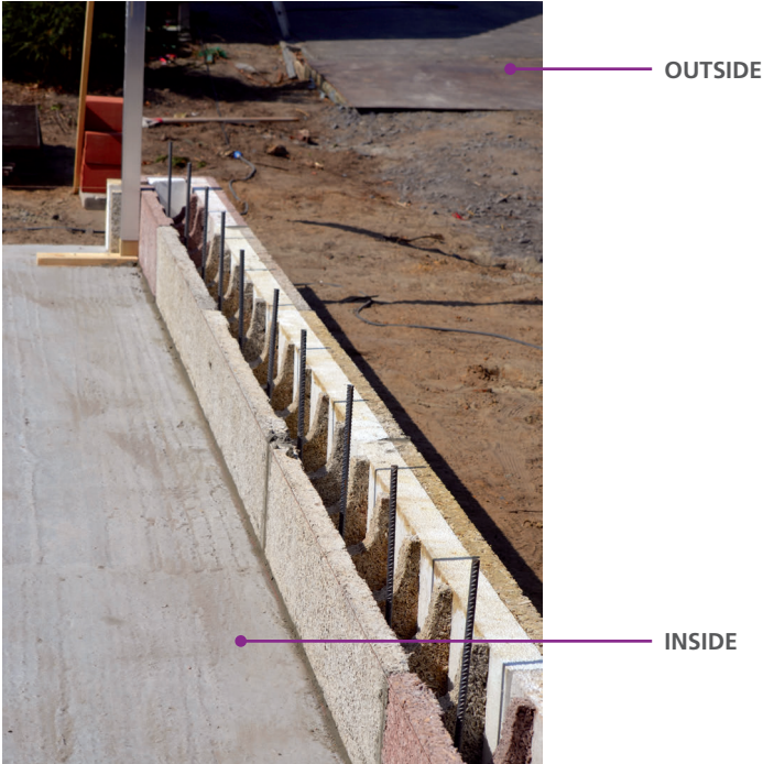
Figure 6.7 Lay blockwork to create formwork around steel reinforcement.
