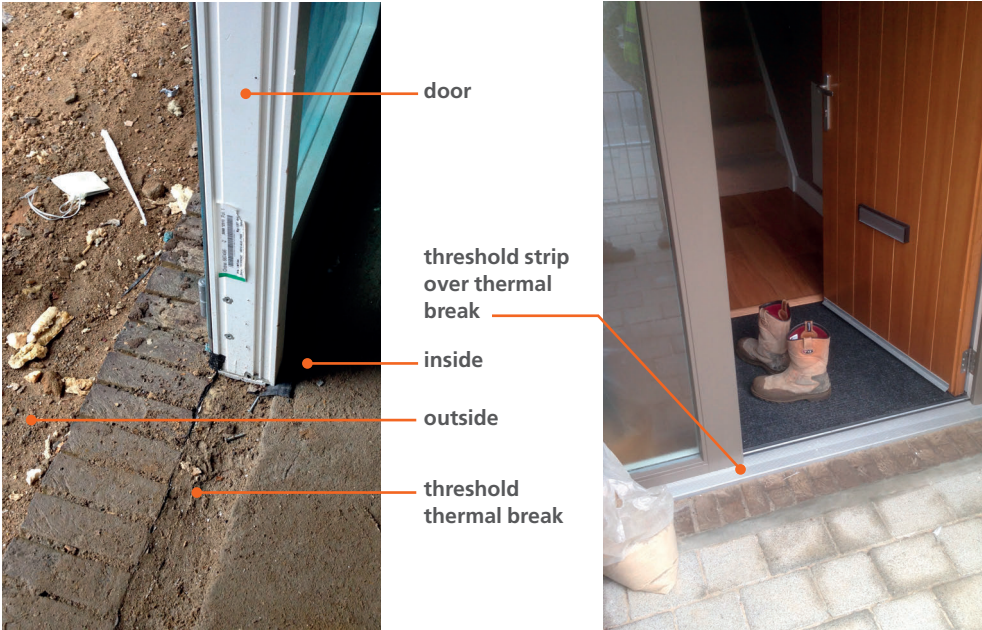
Figure 4.15 Door threshold before doorset is fitted (left).
