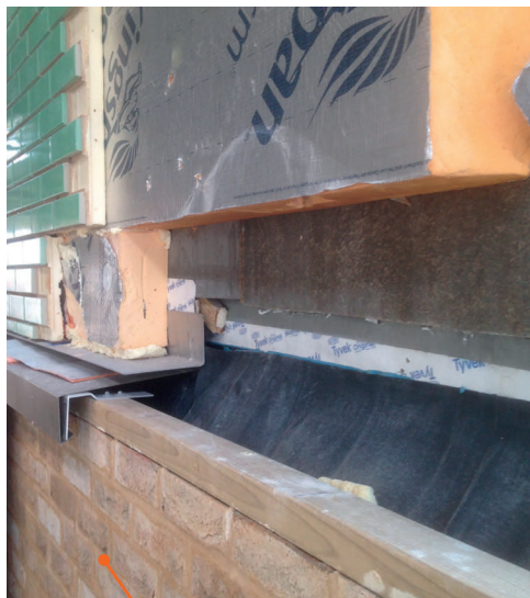
Figure 4.22 Continuous insulation at junctions and up to windows and doors (right).
