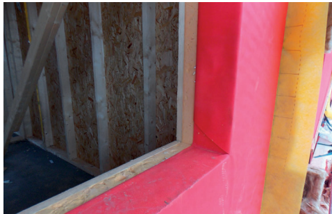
Figure 5.18 SIP window opening from outside (top left).
