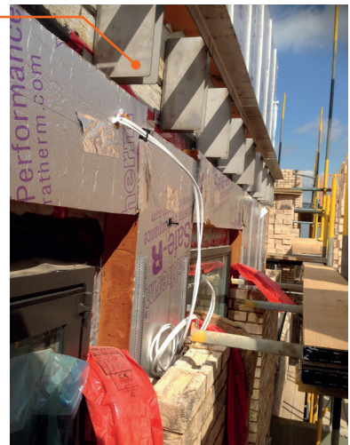
Figure 4.8 Shelf angles used to support brick.
