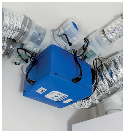
Figure 8.30 a & b MEV unit installed with demand control.
