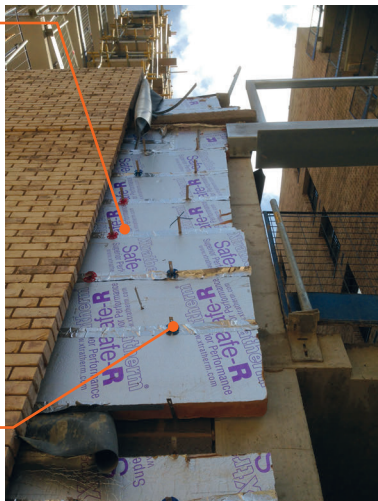
Figure 4.8 Shelf angles used to support brick.
