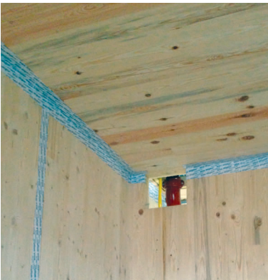
Figure 7.6 CLT is vulnerable to moisture and so needs to have a concrete or masonry upstand and other significant damp-proof detailing (below right).
