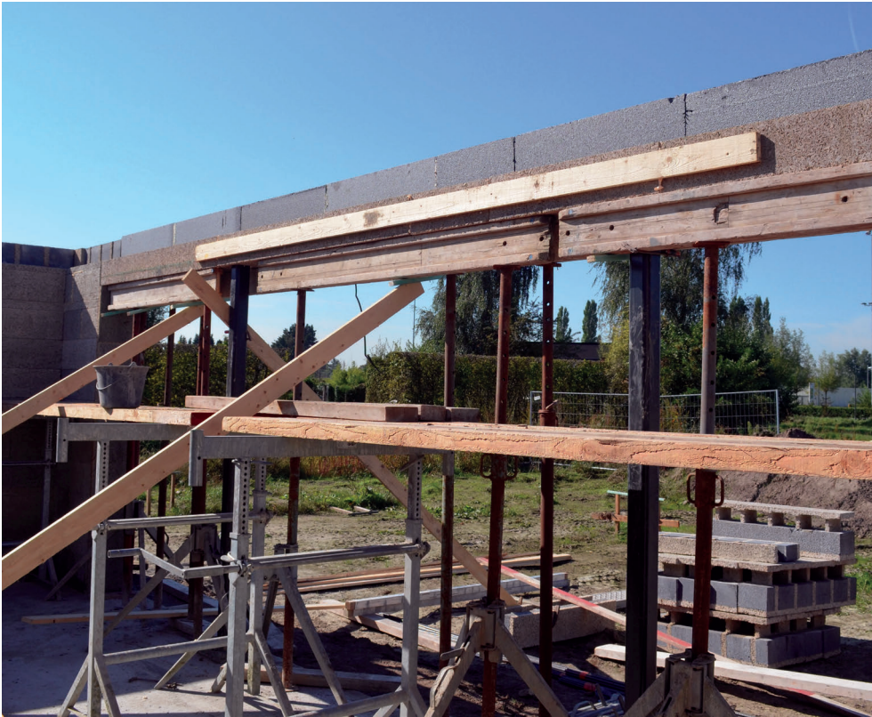
Figure 6.17 Large door opening – lintel and temporary support (left).
