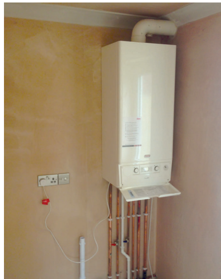
Figure 8.9 a & b Combi boiler with flue gas heat recovery.
