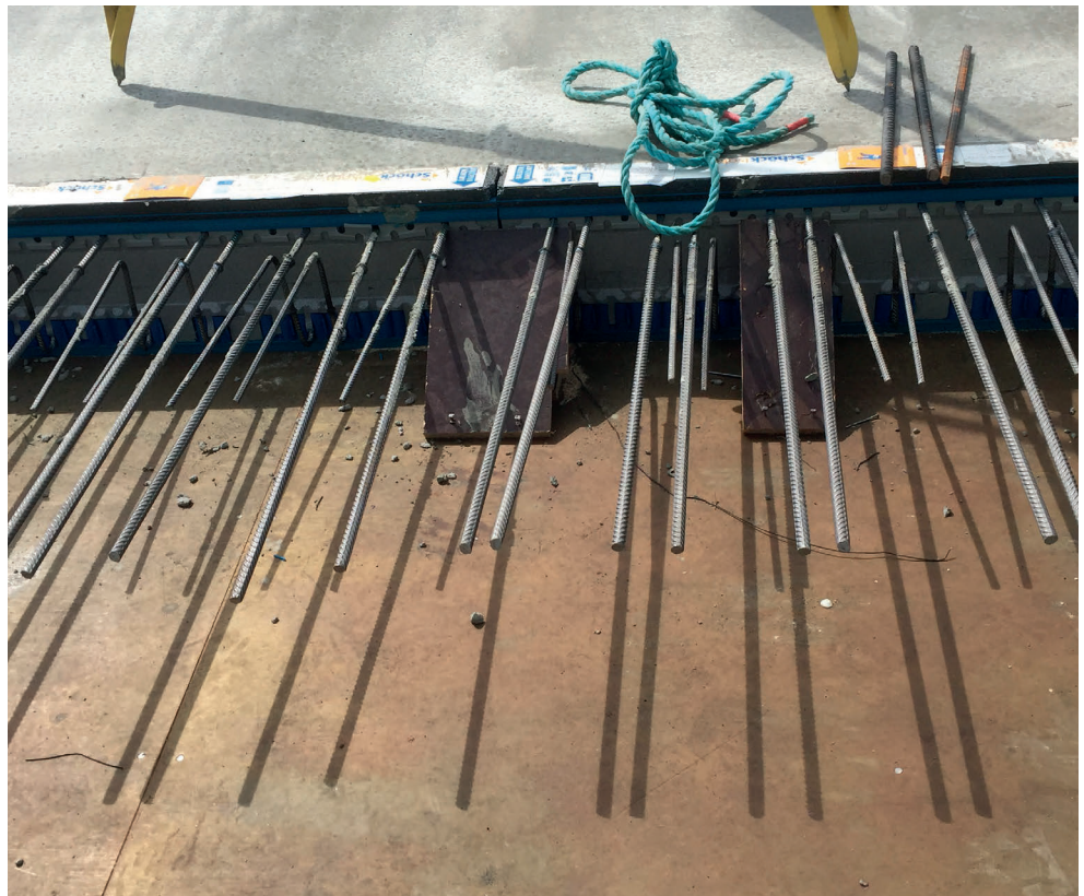
Figure 4.30 Thermal break being installed to separate cantilevered balcony.
