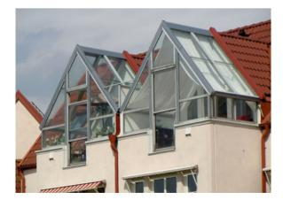
**Fig. 13.10** Example of sunspace integrated with the building structure
