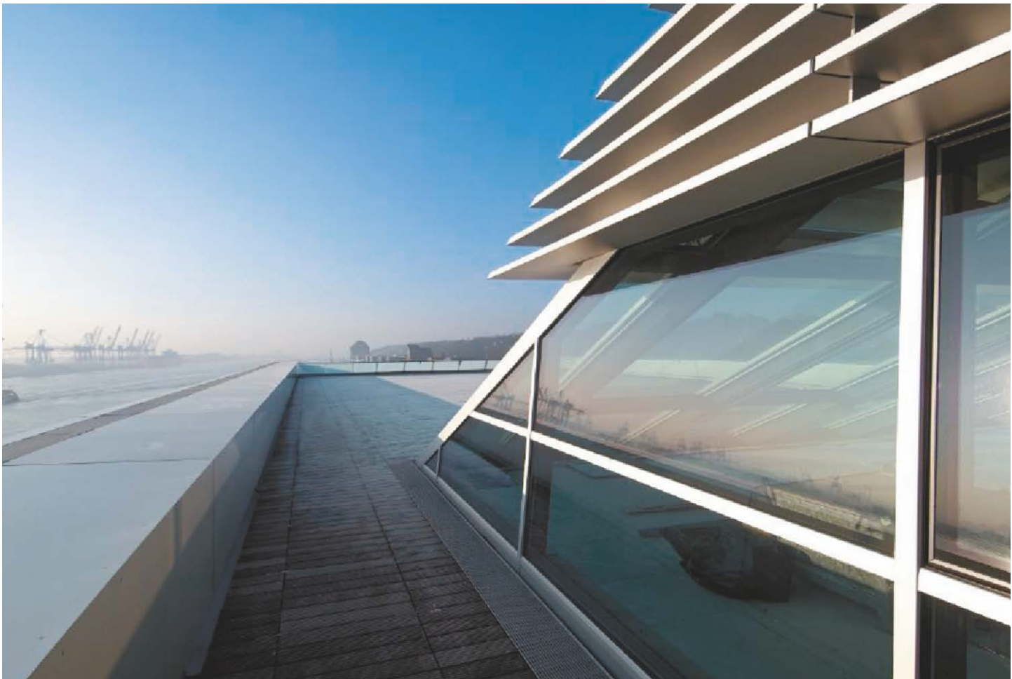
Fig. D1.10 View from the Dockland building roof
