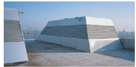
Fig. D1.8 Recooling unit as »ship funnel«
