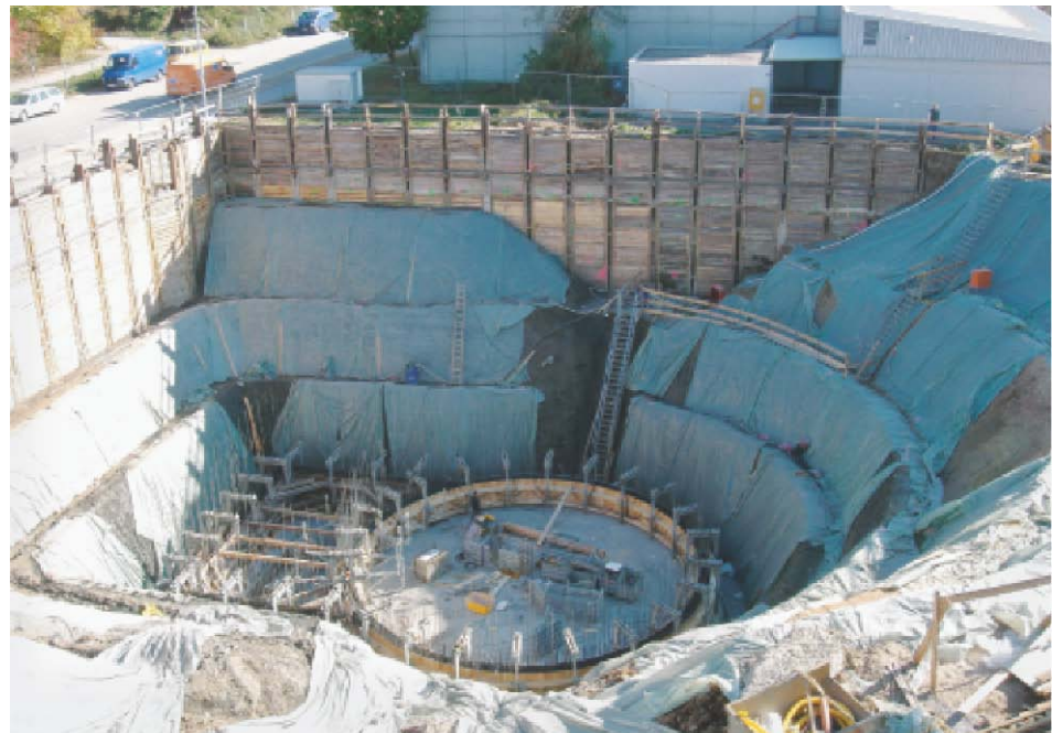
Fig. C2.24 HUK Coburg – Construction of 1100m 3 sized sprinkler/cold water storage
