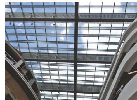
Fig. D8.6 A photovoltaic system was integrated into the glass roof.
