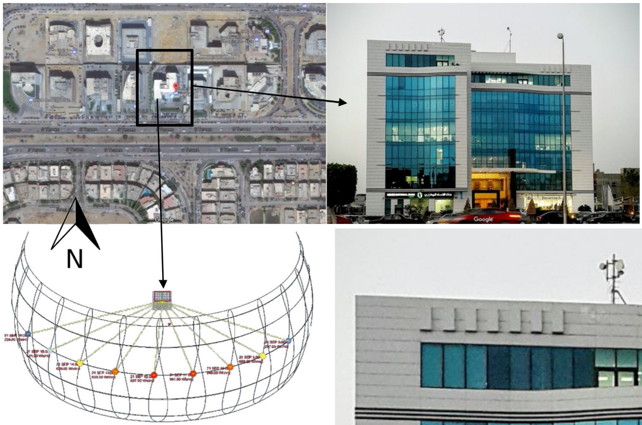
Fig. 1. (Top left) Location of the office building at the 90th street in New Cairo, Egypt [25], exported from Google Earth. (Top right) The image of the office building, Union National Bank UNB in Egypt [26]. (Bottom left) Sunlight directions, exported from Grasshopper. (Bottom right) Close view to the office room.
